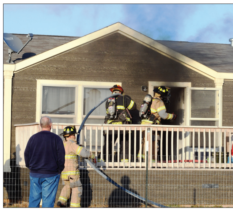
SMOKE DAMAGE — Firefighters work a structure a fire on Private Road 4219 near Decatur Tuesday night.
